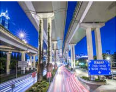
Infrastructure in Japan
